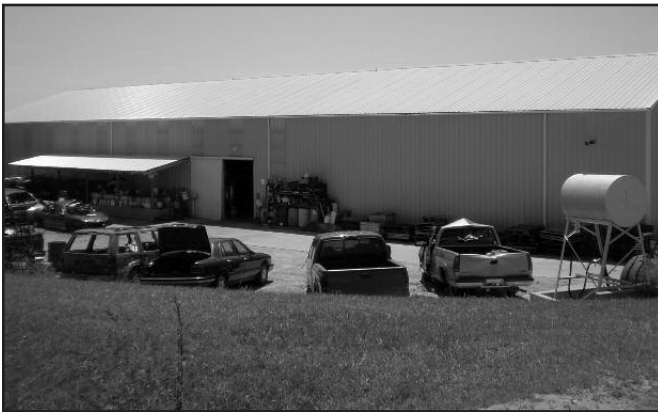
Tear down building and motor storage
